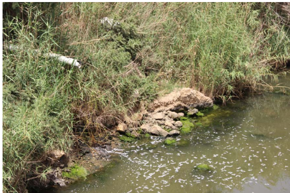
Figure 12: Discharge of waste water in the Oustouan River (the pipe of discharge appears clearly).
