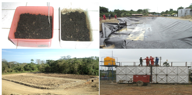
Figure 5: Bioremediation method of oily sludge contaminated soil from lab scale microcosm (upper left) to field scale application i.e. geomembrane lining process (upper right); typical bioremediation cell (lower left); augmented microbe seeding tank (lower right).
