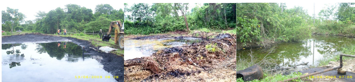
Figure 1: Untreated oily waste from abandoned sludge pit (left), rising oily waste originally from oil sludge burial site (middle), and abandoned drilling pits (right). (author's project documentation with permission from LAPI-ITB Consultant).
