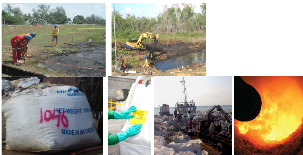
Figure 2: Co-processing of oily sludge activities from (upper left to lower right) site characterization-excavation-containment-labelling-transportation-and thermal destruction in cement kiln. (author's project documentation with permission from LAPI-ITB Consultant).
