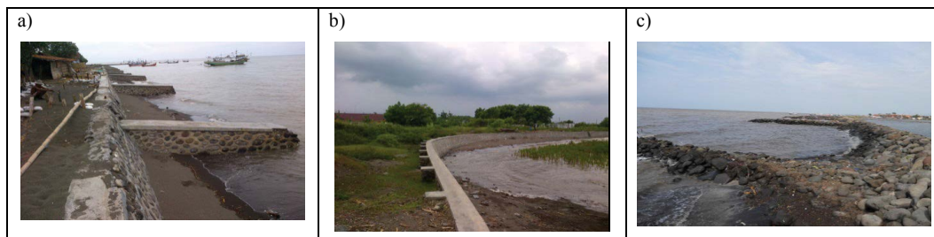
Figure 6a: Embankments and groin with stone cement, b. Embankment without groin and stone cement, c. Embankments and groin with stone crevices.
