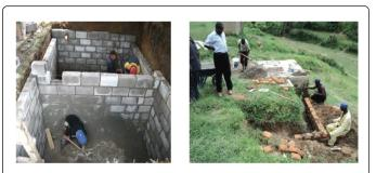
**Figure 5**: (a) On the left, the building process of the designed septic tank for a selected primary school of 150 students (b) on the right, the completed septic tank.
