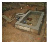
**Figure 4**: (a) On the left, the building process of the designed septic tank for 8 occupants household and (b) on the right, the final stage.
