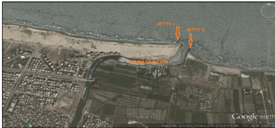
Figure 2: Gamasa drain and two constructed jetties.
