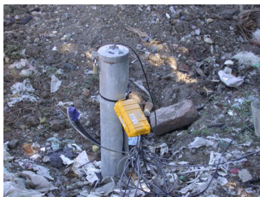
Figure 3: Piezometer tube completely protected with metal casing.
