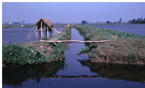
Figure 3: Central sewage canal fed to different Bheris.
