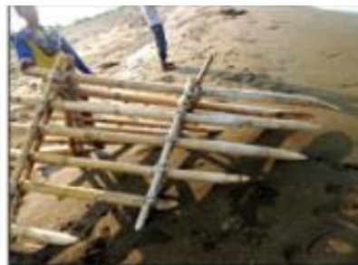
Figure 7: Coastal protective devastated on Karang Dempel sandbars Sub District of Losari and on Randusanga beach Sub District of Brebes.
