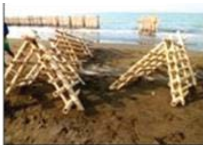
Figure 7: Coastal protective devastated on Karang Dempel sandbars Sub District of Losari and on Randusanga beach Sub District of Brebes.
