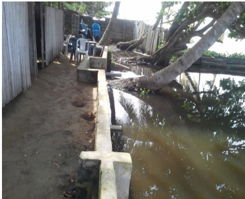
Figure 11: Toilet drains released into water.
