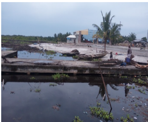
Figure 5: A multi-million-naira town hall in Makun community. The land on which the building is erected is reclaimed from the creek. Source: Author's Fieldwork, 2018.
