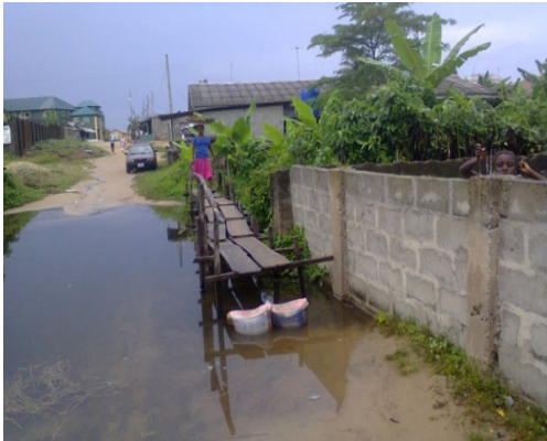
Figure 4: Flooded minor road in Ibereko community (Badagry) Lagos. Source: Author's Fieldwork, 2018.
