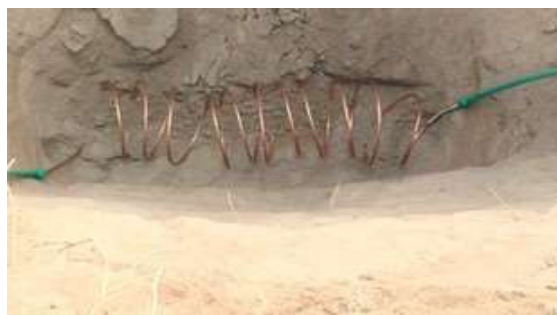
Figure 2: Buried copper coil at 14 ft. depth.
