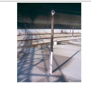
Figure 2: The deck leg of storage tank.
