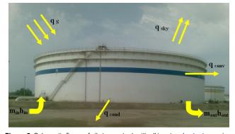
Figure 5: Schematic figure of oil storage tank with all input and output energies.
