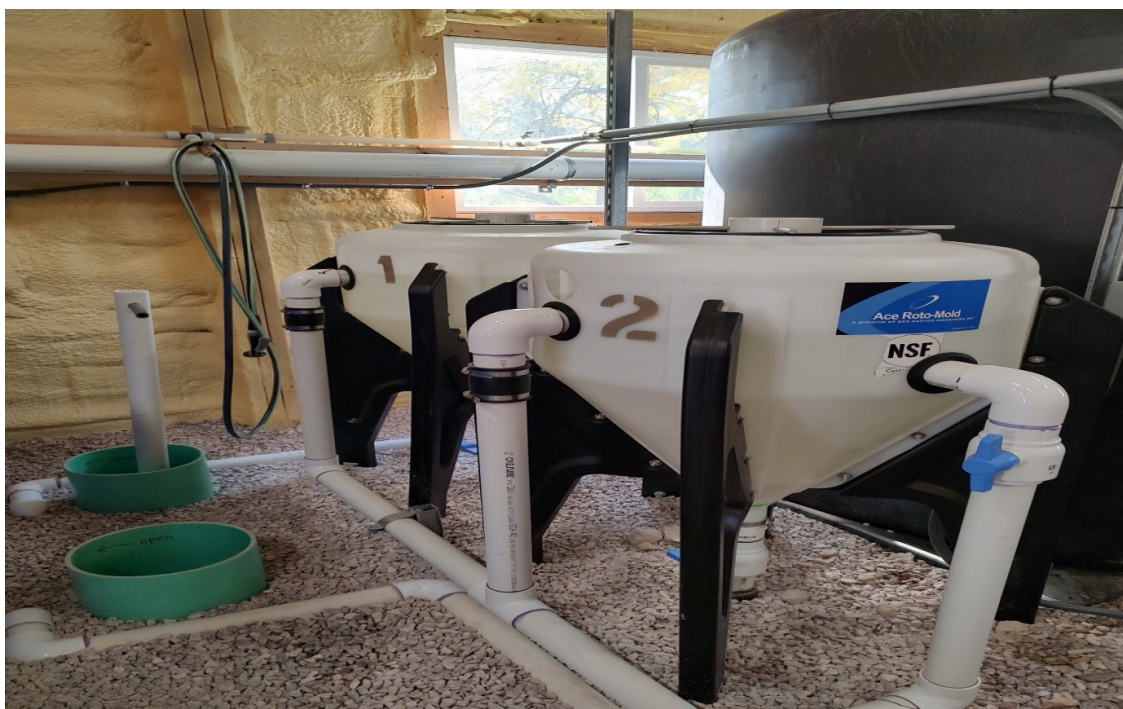
Figure 5: External view of inductor tank used to build a Radial Flow Settling (RFS) tank.
