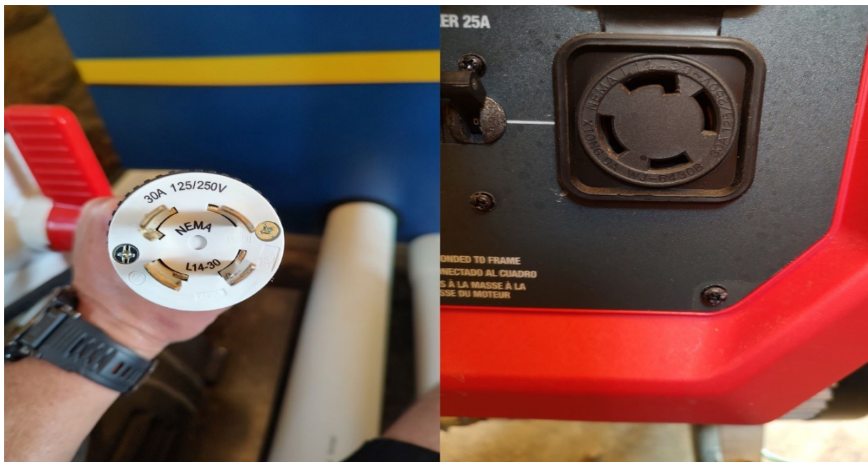
Figure 16: NEMA L14-30 plug and generator receptacle used for emergency operation of the main system pumps.
