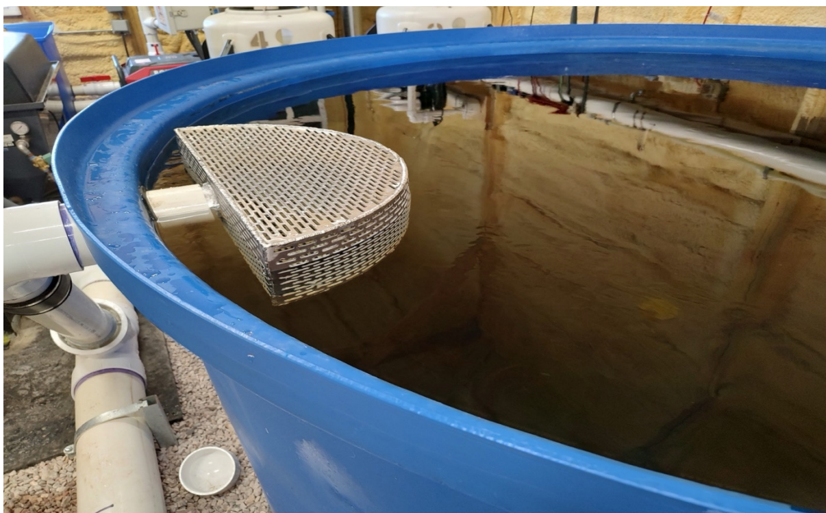
Figure 2: Culture tank top drain perforated aluminum structure.
