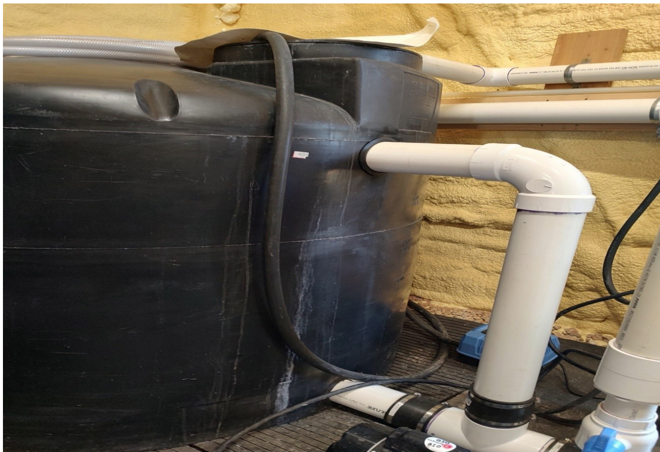
Figure 7: Overflow protection drain for Moving Bed Bioreactor (MBBR).
