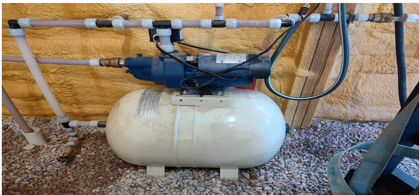
Figure 11: Shallow well jet pump and pressurized tank used to keep water reservoir filled.
