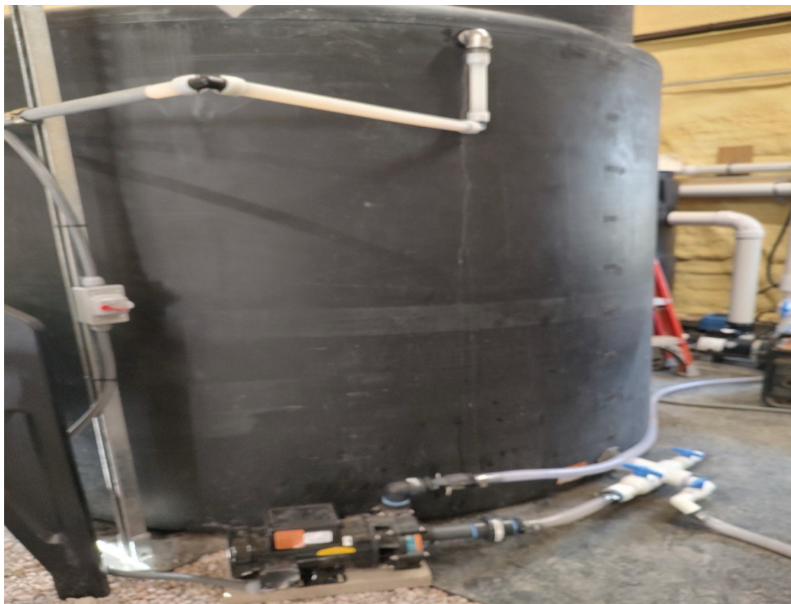
Figure 12: Water reservoir with ¼ HP pump used to supply water to the system.
