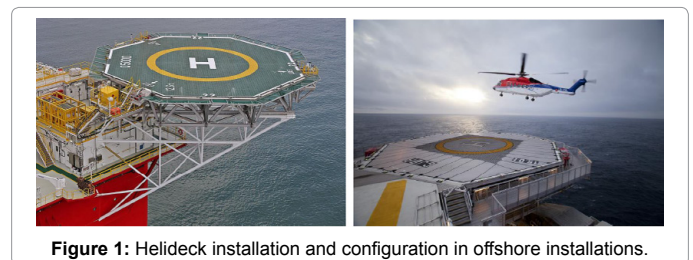
Figure 1: Helideck installation and configuration in offshore installations.
