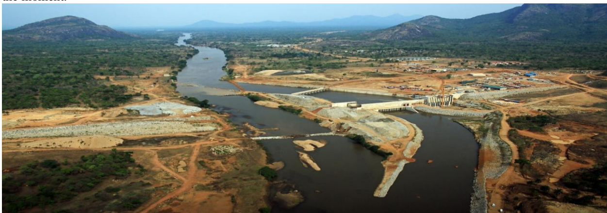
Fig. Kashimbilla Multipurpose dam Project
