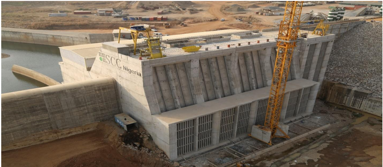
Fig. 4 Kashimbilla Multipurpose dam under construction
