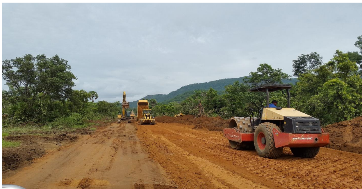
Fig. 8. Construction of access road to affected communities
