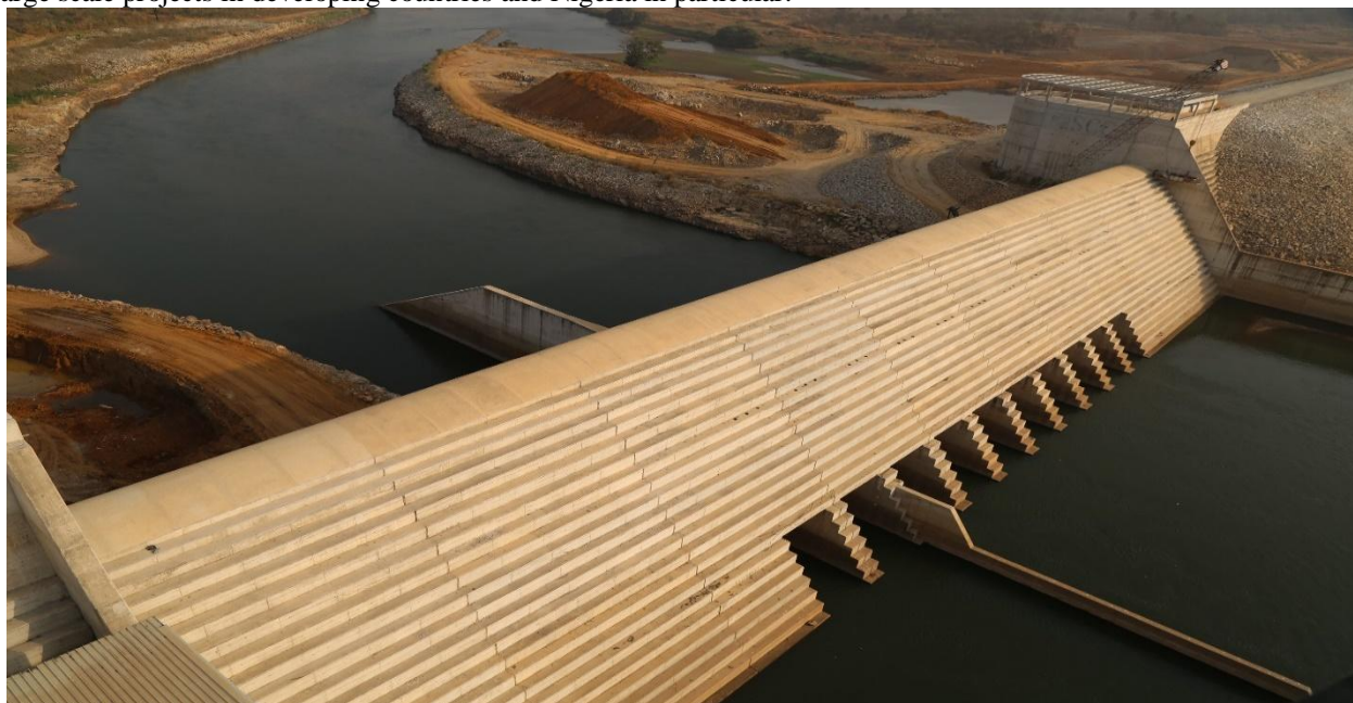
Fig. 3 Constructed embankment of Kashimbilla Multipurpose dam
