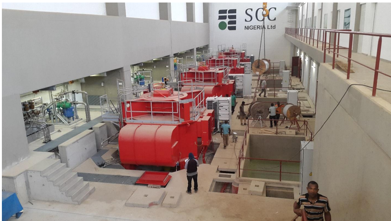
Fig. 7 Turbines at the Kashimbilla Multipurpose of dam
