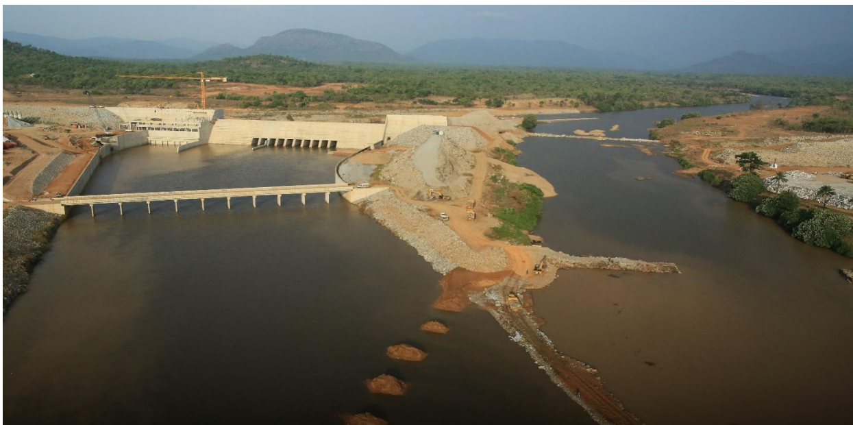
Fig. 2. Kashimbilla Multipurpose dam and spill way
