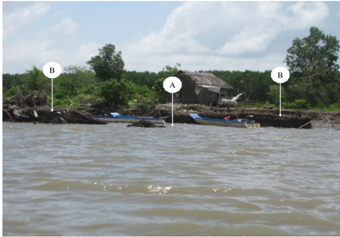
Figure 6: Abandoned pond in An Bien district, with breached dykes; (A) Pond area; (B) Breached dykes.
